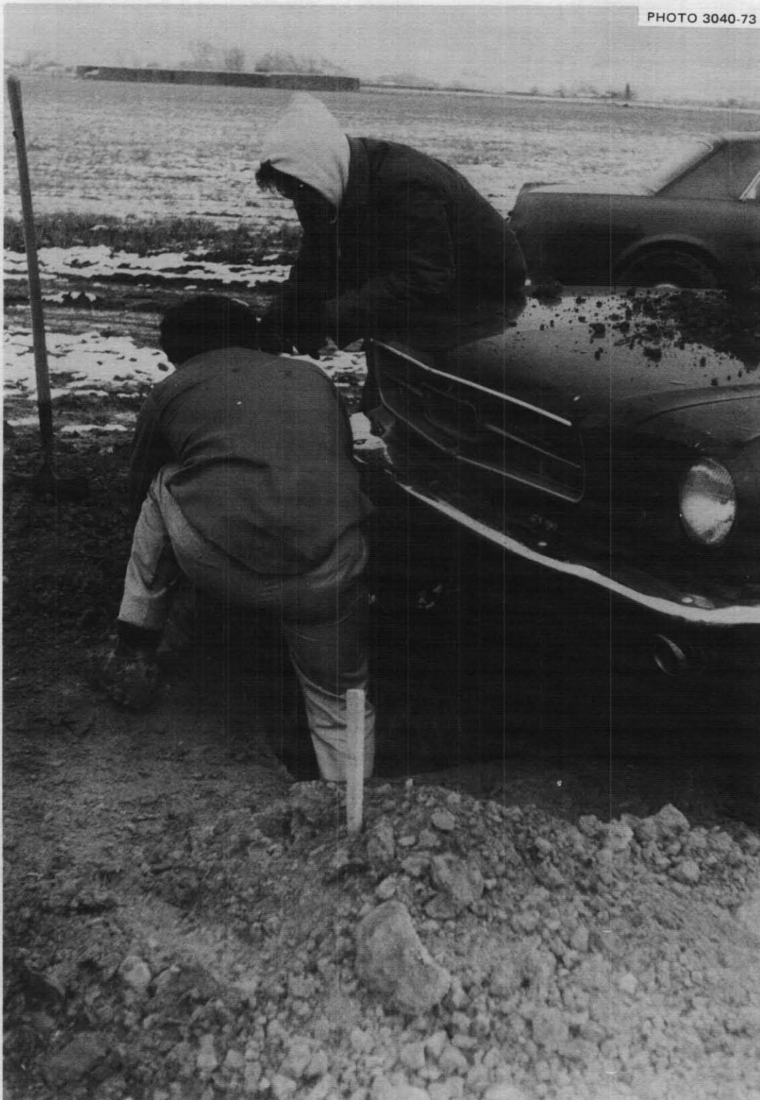
Fig. 6.13. Placing earth-filled plastic garbage bags around the edges of the entryway trench. The mother was able to remain on the site all of the second day and do some work – thanks to a borrowed pair of insulated boots that kept her feet from getting painfully cold.
